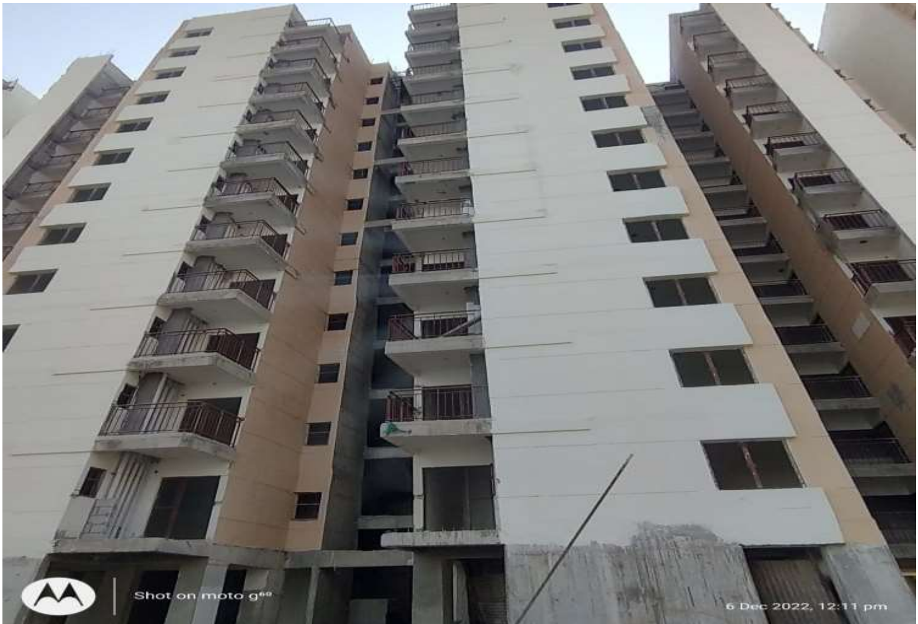
2BHK Tower 2B/T6 internal & External paint work in progress.
