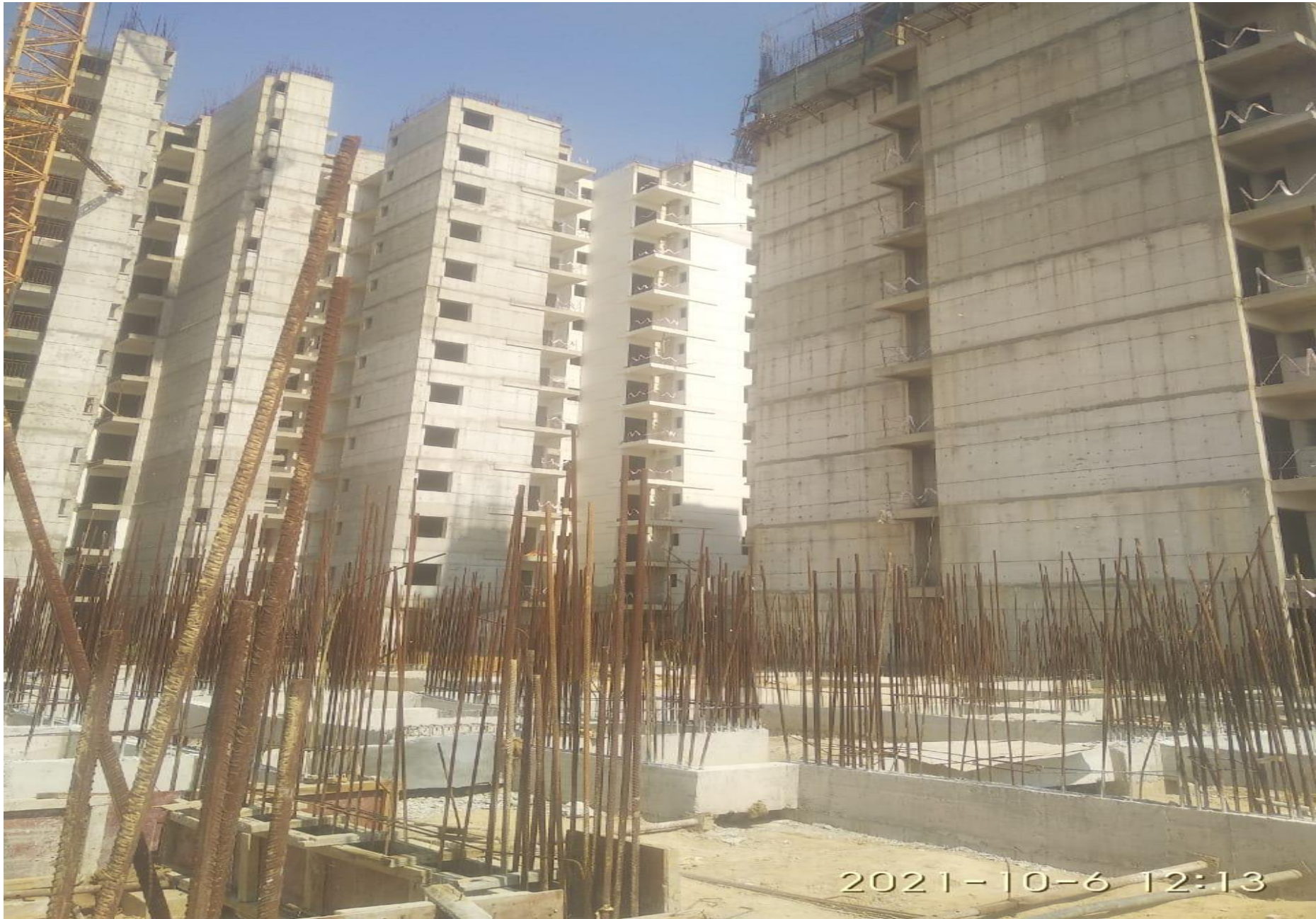
2BHK Tower 2C/T7 External paint work in progress.
