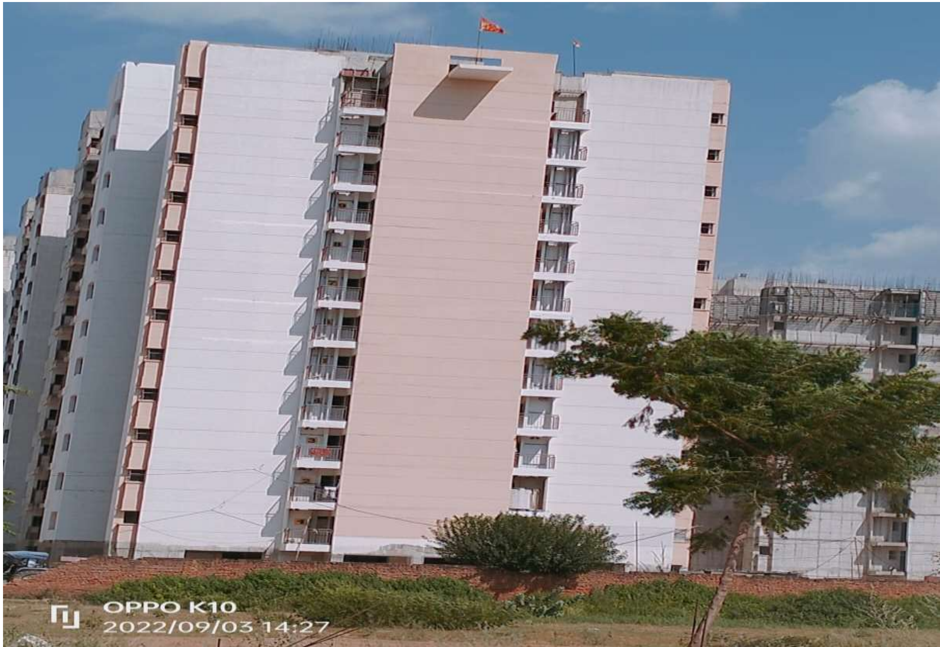
2BHK Tower 2A/T5 External paint work in progress.
