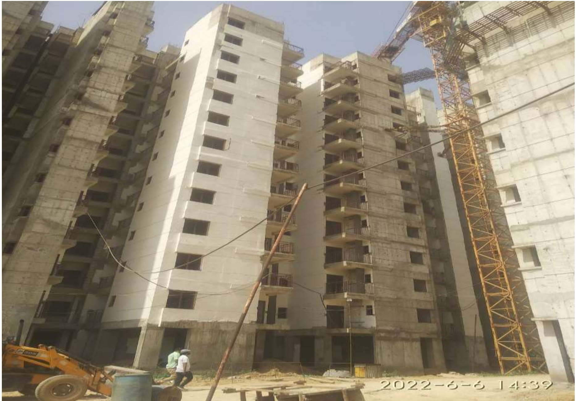
2BHK Tower 2B/T6 internal & External paint work in progress.
