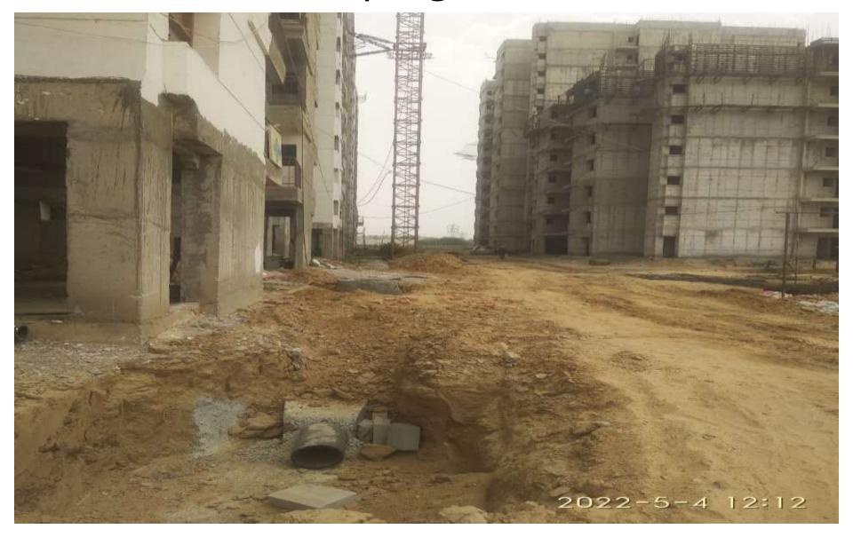
External Sewer Line pipe installation work in progress.
